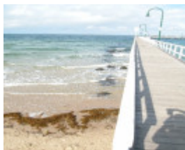
Lagoon Training Walls Wharves And Drain April 2003 Lagoon Pier East Stone 001
