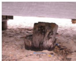
Lagoon Training Walls Wharves And Drain Port Melbourne April 2003 Lagoon Pier Pile 002
