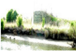
Explosives Factory Bridge Abutment Maribyrnong June 2003
