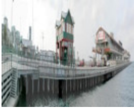
Station Pier Port Melbourne July 2003 001
