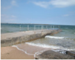
McGregor Street Drain Culvert Port Melbourne March 2003
