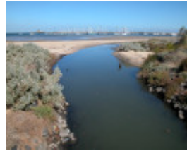
Cowderoy Street Drain Culvert Williamstown April 2003 Drain Piles 002
