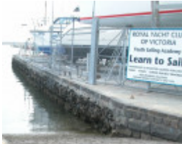
Jacks And McIntosh Boat Repair Facilities Williamstown Aug 2003
