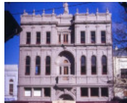
h00987 mechanics institute sturt st ballarat front view she project 2003
