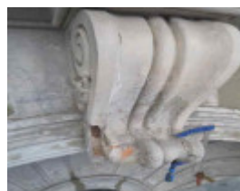
Before Photograph - Reference F3924 2014
