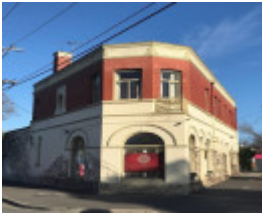
68-70 Armadale Street, Armadale
