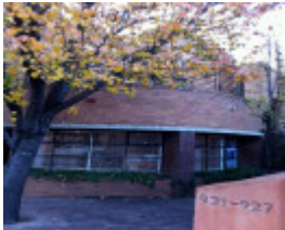
Flats & shops, 921 High Street
