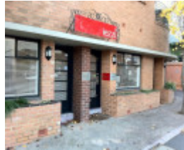
Flats & shops, 921 High Street
