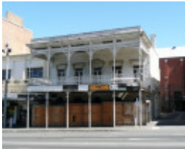
FORMER UNICORN HOTEL FAÇADE AND VERANDAH SOHE 2008
