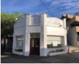
8 Morey Street, Armadale
