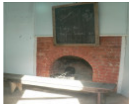
Gringegalgon Soldiers Memorial Hall - rear dressing room
