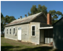
Gringegalgon Soldiers Memorial Hall - viewed from north-west
