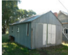
Gringegalgon Soldiers Memorial Hall - supper room/kitchen
