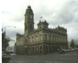
1 ballarat town hall exterior view 1993
