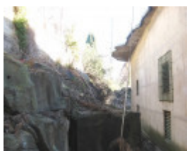
Maribyrnong substation quarry wall at rear
