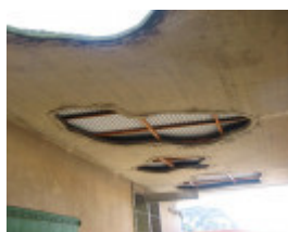
Maribyrnong substation cutouts in concrete roof
