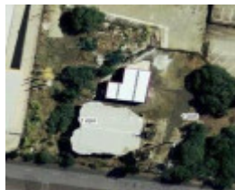
Maribyrnong substation aerial view
