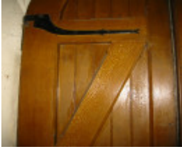
St Andrews Kirk Door Detail 01 Oct 03
