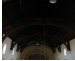
St Andrews Kirk Interior 02 Oct 03
