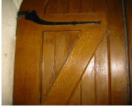
St Andrews Kirk Door Detail 01 Oct 03
