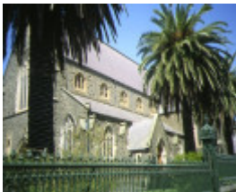
1 st patrick's cathedral ballarat exterior view of cathedral
