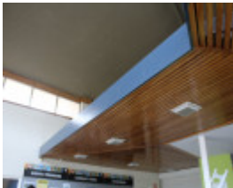
Interior of primary entrance building - timber panelling
