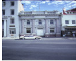
1 former commercial bank of australia bendigo front view
