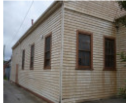
PROGRESS HALL SIDE ELEVATION
