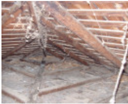
h02085 macedon house gisborne august05 pr 40
