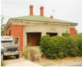
FORMER KAHLAND WINERY & CELLARS SOHE 2008
