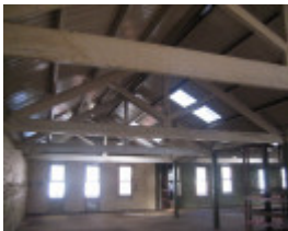
61-9 A'Beckett St first floor MZ 24 05 2007
