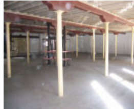
61-9 A'Beckett St ground floor MZ 24 05 2007
