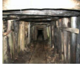
0198 Wonthaggi State Coal Mine Eastern Area Back tunnel incline
