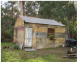
14228_Great Ocean Road Kennett River Hut August 2010 b.jpg
