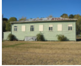
14247 Former Ballarat RAAF Base gymnasium
