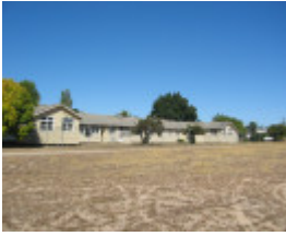
14247 Former Ballarat RAAF Base Admin building
