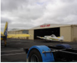
14247 Former Ballarat RAAF base Bellman Hangars
