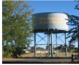
14247 Former Ballarat RAAF Base water tower
