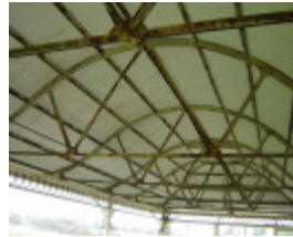
14252 Hamilton racecourse 4Sept06 grandstand roof
