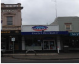
Cold Rock 5 Sturt Street, Ballarat Central
