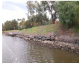
Pipemaker Park Wharf Maribyrnong July 2003 North Section
