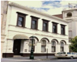
H0403 former bank of nsw view street bendigo
