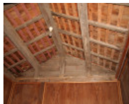
Roof structure - internal view. Mar 2007.
