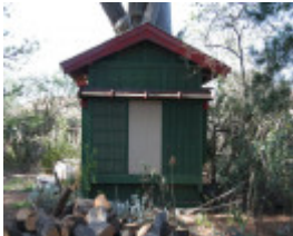
General external view. Mar 2007.
