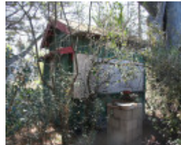
General external view. Mar 2007.
