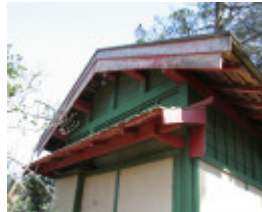
Gable detail. Mar 2007
