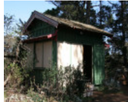
General external view. Mar 2007.
