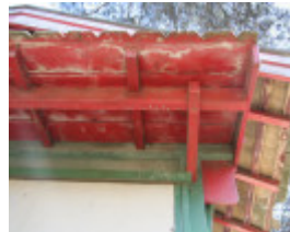
Eaves detail. Mar 2007.
