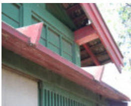
Roof detail. Mar 2007.
