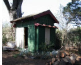
General external view. Mar 2007.
