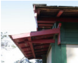
Eaves detail. Mar 2007.
