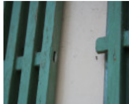
Lattice detail. Mar 2007.
