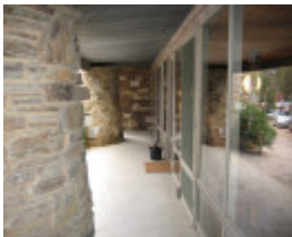
H2118 Baker House Bacchus Marsh verandah detail rc May 2006
