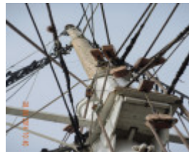
Before Photograph - Reference F3930 2014
