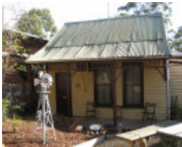
Diamond House_Stawell_timber cottage_Kj_29 may 08
