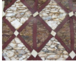
Diamond House- Stawell_detail_KJ_29/5/08
