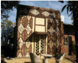
Diamond House_Stawell_garden elevation_KJ_29/5/08
