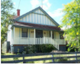
710 Lydiard Street North
