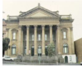
1 masonic hall bendigo front view
