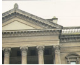
masonic hall bendigo detail pediment
