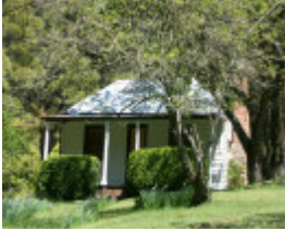
Guggenheimer Historical Cottage, Moorabool Shire Heritage Study Stage 1, 2010
