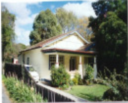
House at Mount Dandenong Rd 272
