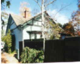
House at 298 Mount Dandenong Rd
