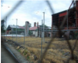
FORMER BENDIGO GAS WORKS SOHE 2008
