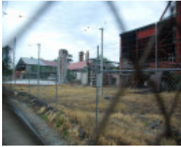
FORMER BENDIGO GAS WORKS SOHE 2008
