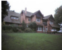
1 edrington berwick front view of house apr1985
