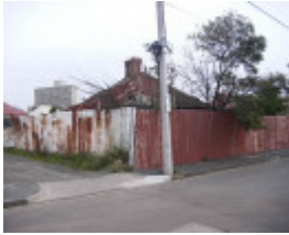
43 Aitken Street WILLIAMSTOWN, Hobsons Bay Heritage Study 2006
