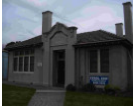
Altona Primary School No. 3923 Complex and trees, Hobsons Bay Heritage Study 2006 - The image shows the 1922 entrance
