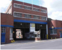
Melbourne Glass Bottle Works (former), Hobsons Bay Heritage Study 2006
