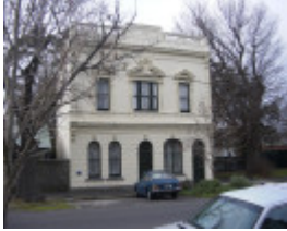
George Hotel (former), Hobsons Bay Heritage Study 2006
