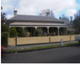
135-137 Cecil Street, Hobsons Bay Heritage Study 2006
