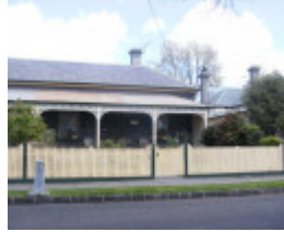
135-137 Cecil Street, Hobsons Bay Heritage Study 2006
