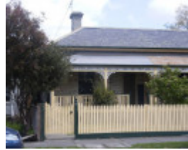
135-137 Cecil Street, Hobsons Bay Heritage Study 2006
