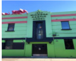
89 Albert Street, Windsor
