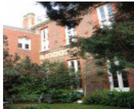
Alfred Hospital Aug 26 2011 KJ east side.jpg
