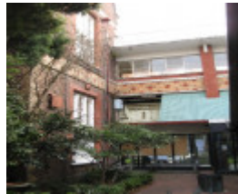
Alfred Hospital Aug 26 2011 KJ east side.jpg
