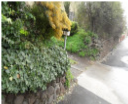
811 Sydney Rd - retaining wall
