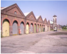
Newport Railway Workshops (former), Hobsons Bay Heritage Study 2006
