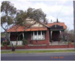
Newport Railway Workshops Deputy Manager's Residence (former), Hobsons Bay Heritage Study 2006
